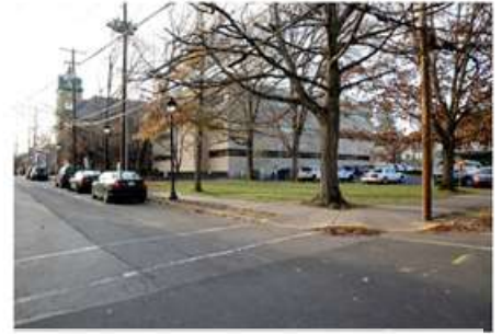
Monroe County Courthouse, Stroudsburg, PA.
